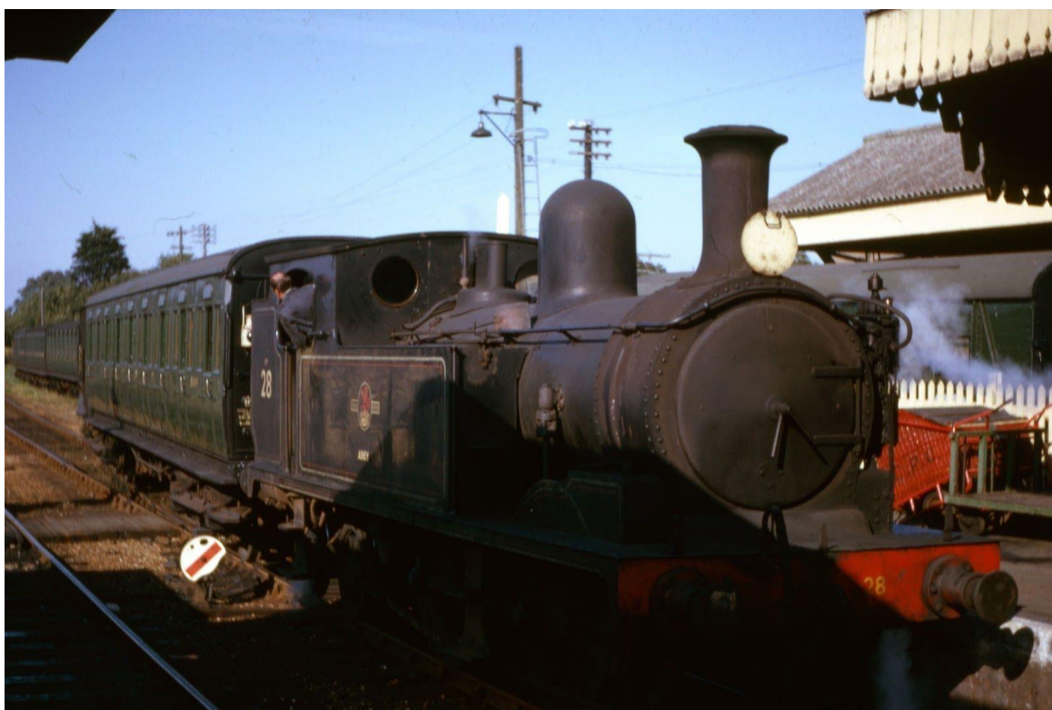
Isle of White 1966: An ageing LSWR O2 0-4-4 tank engine, W28, 'Ashey' with fireman awaiting the right away perhaps with the driver in the auto coach. Built at Nine Elms in 1890 and moved to the IOW in 1926 this venerable little loco was withdrawn in 1967 when the Island Line was electrified and the ex-Underground trains moved there. Thanks to Gordon Woods for scanning the original colour slide.
